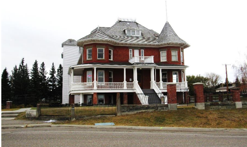
General view of the Site building.
